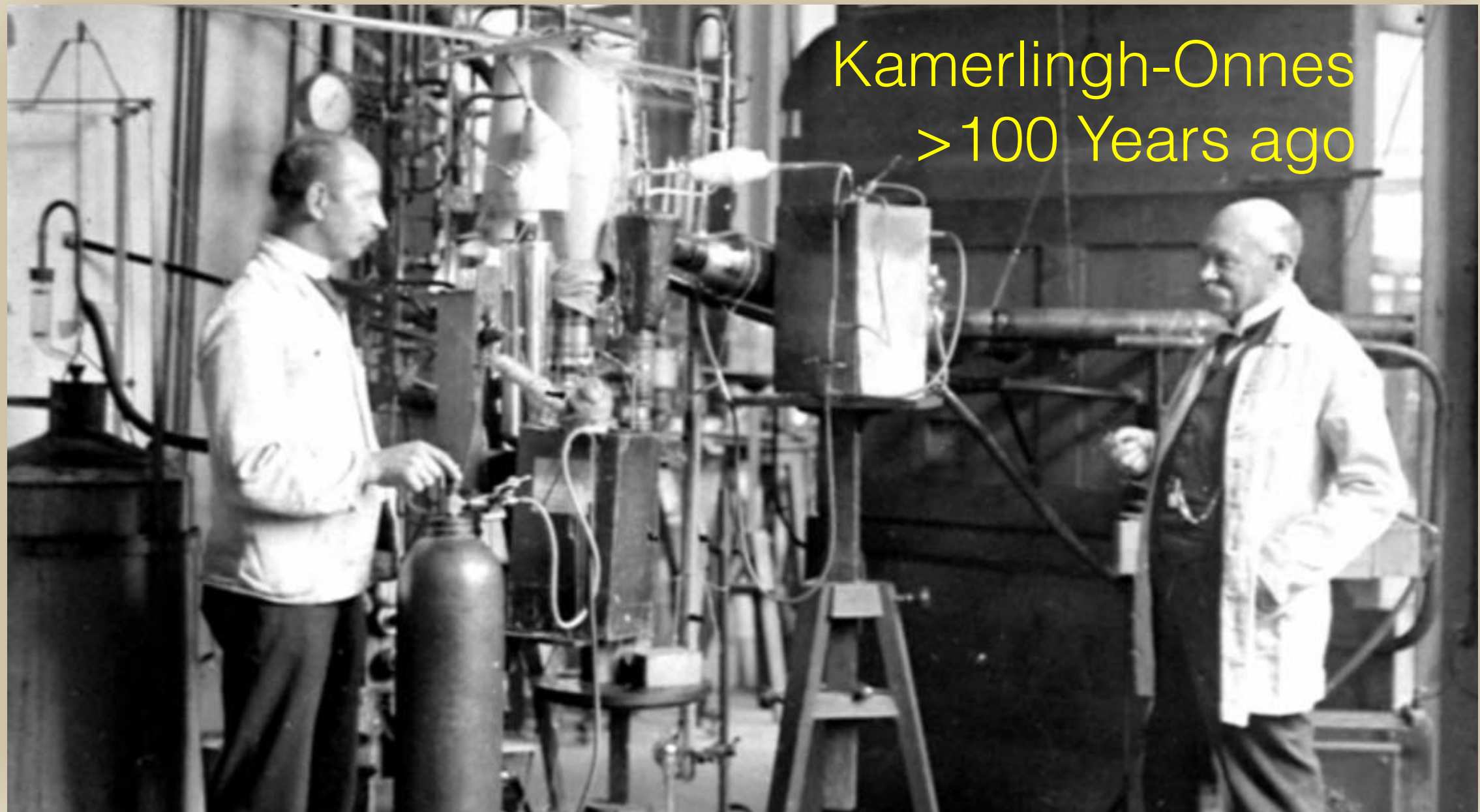
Figure 1. Heike Kamerlingh Onnes (right) and Gerrit Flim, his chief technician, at the helium liquefier in Kamerlingh Onnes's Leiden laboratory, circa 1911.
